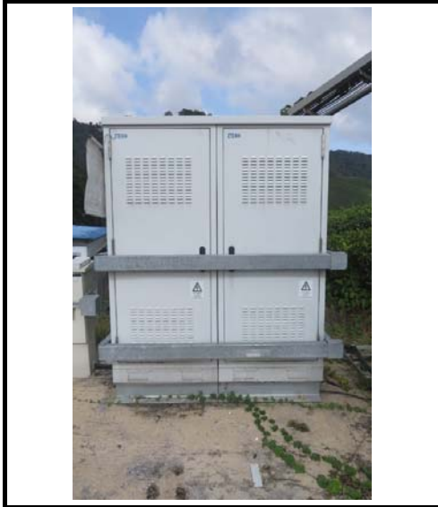
Existing RBS #1 Location (Full View)
