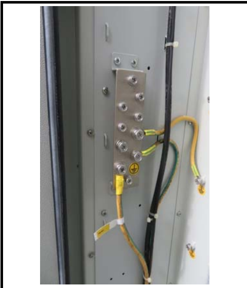
Existing MGB Location (Inside / Outside Cabin)
