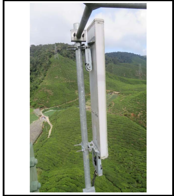
Existing Antenna 1 Sector 3 Zoom
