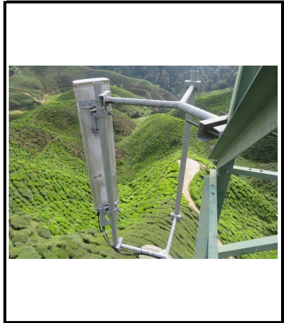
Existing Antenna 1 Sector 1 Zoom
