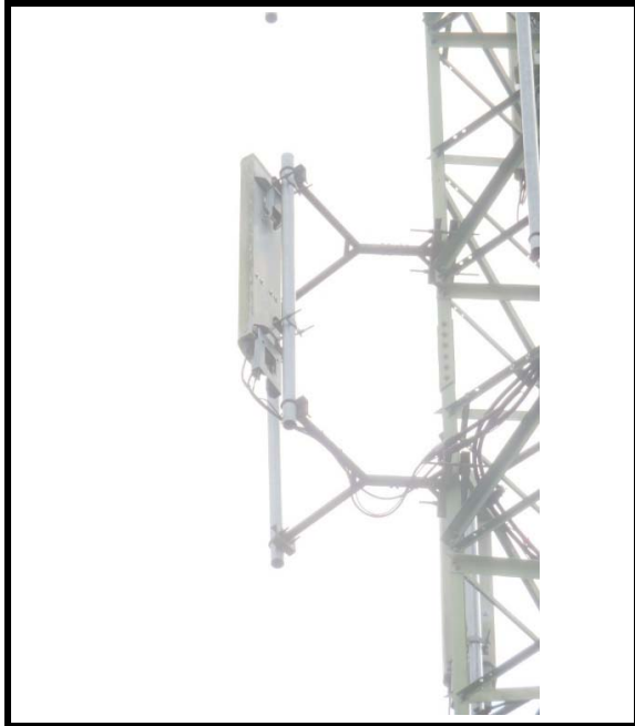
Existing DB HH Antenna (U21) @ 18m AGL, Sector 2
