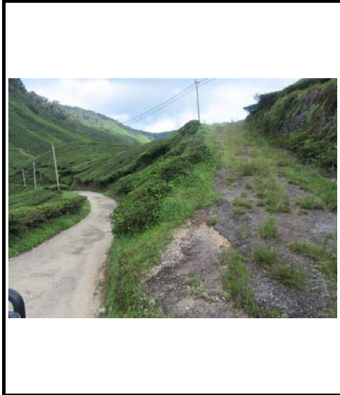
Site Access View 1
