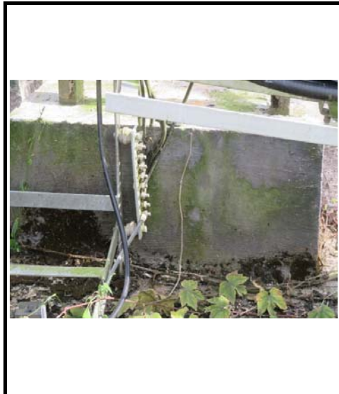
Existing MGB Location (Tower Leg)
